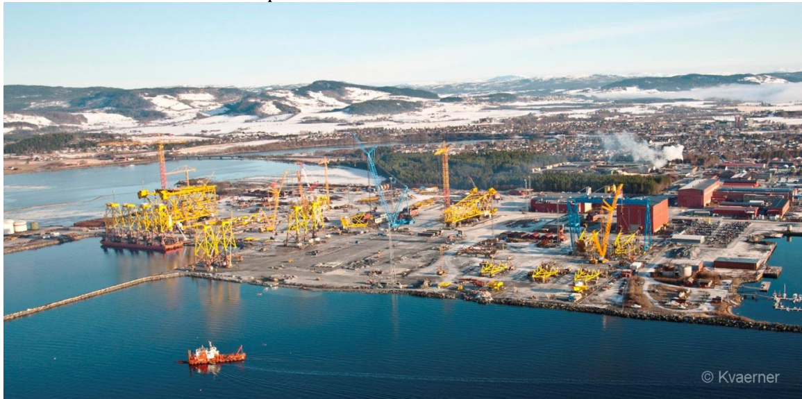
Figure 7: Kværner yard in Verdal.
