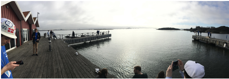
Figure 8: The harbour and test facility area at Volvo Penta
